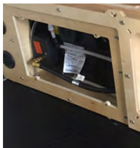
cover plate removed
