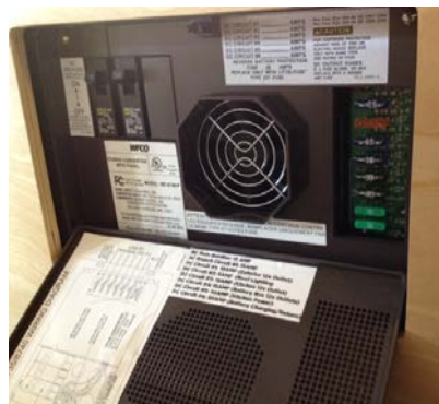
WFCO power center
