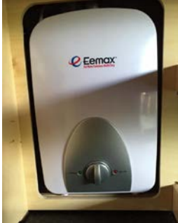
Electric HW Heater
