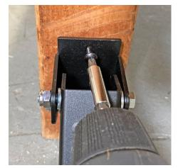
**4.** Drive the top screw in place, then check that the mounting plate is straight, pilot the second hole and add the second screw.
