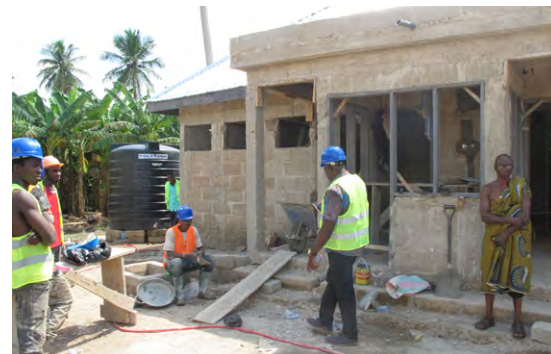
Image: Construction of a new sanitation block in Ashanti, Ghana
