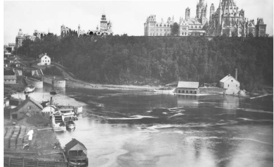
Note the commissariat building to the right of the locks, now the home of the Bytown museum.
