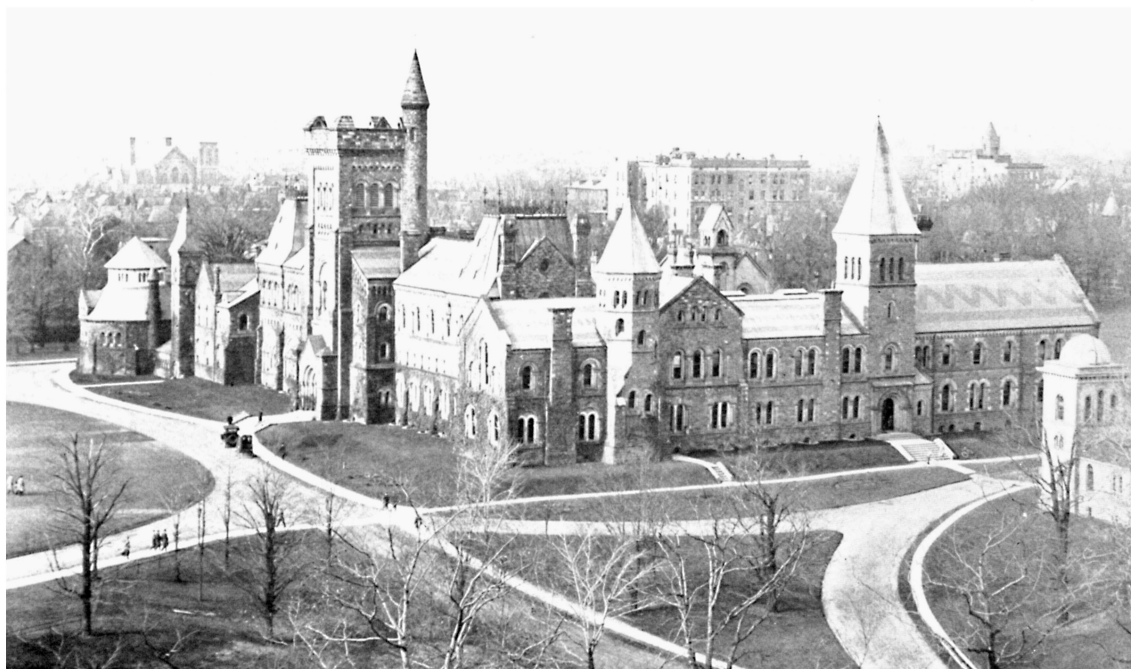
BIRDSEYE VIEW OF MAIN BUILDING
