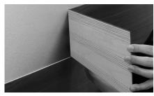
**TIP:** To help ensure an absolute straight starter line with the first plank, we recommend you tap 1 ½" finish nails halfway into the wall along the starting line at every 12". The protruding nails will help position the starter planks along the starting line before they are adhered to the wall. This procedure will not be possible when installing over a block wall. Use extra caution to ensure your first row is straight if you are not able to use nails as a guide.
