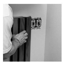
**Step 9)** Installing the top and bottom rows. When installing your top and bottom rows, the planks can be cut lengthwise by using a jigsaw or table saw.
