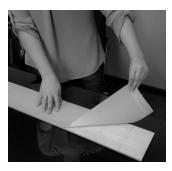
**Step 7)** Cutting the planks. Planks can be cut to fit by using an electric jig saw, miter saw or table saw. It is beneficial to have a sanding block handy to smooth the cut slat edges.
