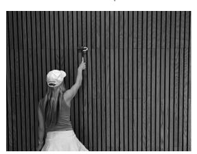
**Step 11)** IMPORTANT! Secure your Acoustic Wallplanks with the included Acoustic Wallplanks Screws with a power drill at the indicated locations.
