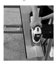
**Step 8)** Unique cuts. Mark locations of light switches, electrical outlets and air vents on the planks before removing the paper liner on the tape. Cut and trial fit *before* removing paper backing — so that you can test your cut plank before adhering it to the wall. These cuts can be made using a drill to create a starter hole if necessary and then cutting with a jigsaw or scroll saw. Additional felt can also be used to border the outlet.
