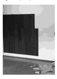
**Step 11)** IMPORTANT! To help set the Vacuubond™ adhesive after the installation is complete, the wall must be rolled using a J-roller to insure the bond. Not using a J-roller can lead to failed adhesion. J-rollers are available for purchase at www.wallplanks.com. If a trim piece is used to finish installation, it can be installed now. Refer to Step 3 for trim installation instructions.
