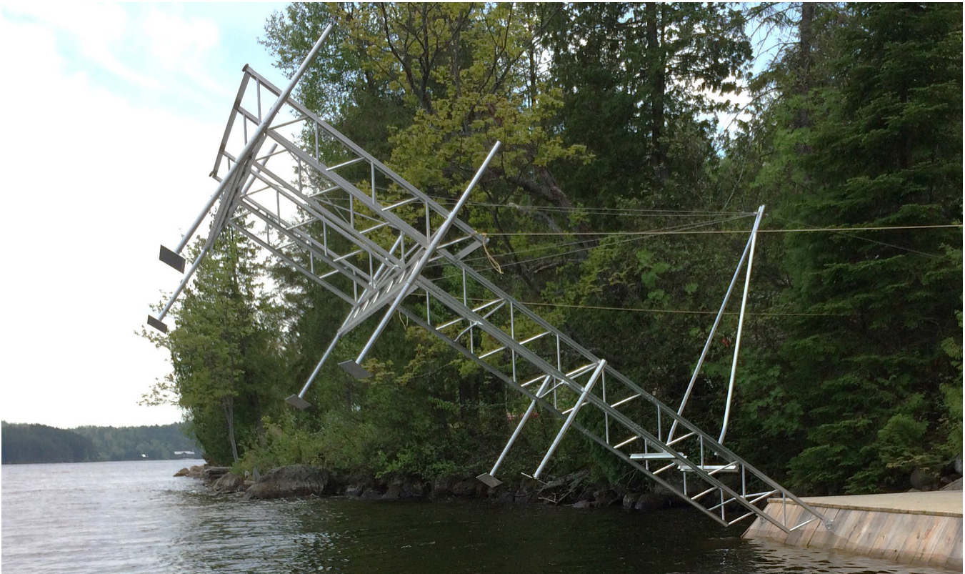
Cantilevered 24' long assembly with 8' x 12' Truss deck incorporated at the end.
