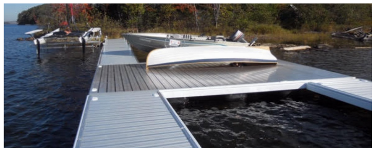
Frame docks from shore connected to Floating dock ramp and floating dock
