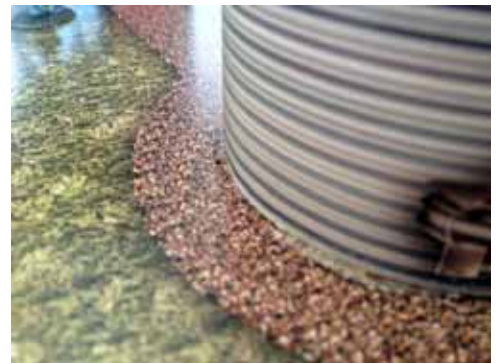
Close-up detail view
