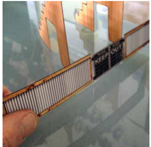
Figure 15 - Attach the rear bleacher fence.
