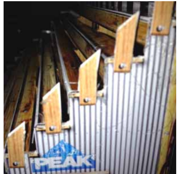
Figure 9 - Attach the handrail supports.
