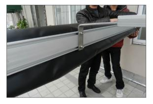
Fix the awning to the mounting brackets with M6 bolts.
