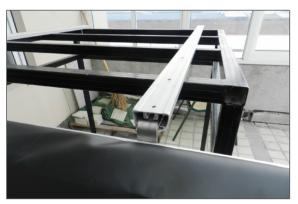
Make sure the awning is the right way around. Use two persons to lift it in place and fix the bolts at the back of the mounting plate to the mounting brackets.
