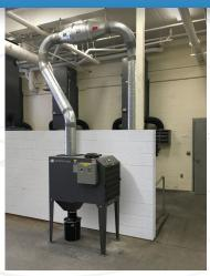
DFC Small Cartridge Dust Collector with hopper
