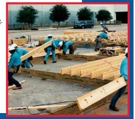
"In working with contemporary homes, building with components holds your dimensions plumb, square and true, ensuring a dimensionally accurate home, reducing call-backs."
