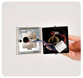
2. Connect the lamp wires with the reserved wires
