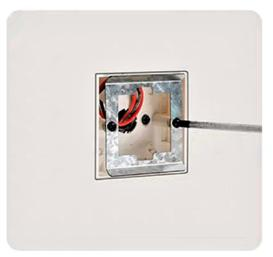
1. Drill holes in the wall according to the size of the lamp base, embed the base into the wall, and secure it with screws
