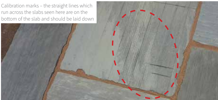
The white marks seen here are characteristic signs of saw marks
