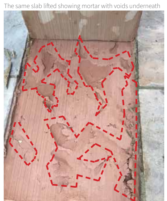
The same slab lifted showing mortar with voids underneath
