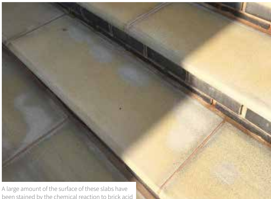
Rectangular beige marks on the slabs here are characteristic of chemical reaction
