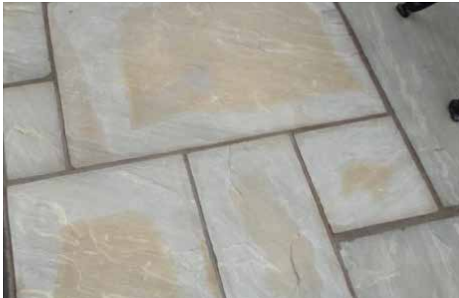
Rectangular beige marks on the slabs here are characteristic of chemical reaction
