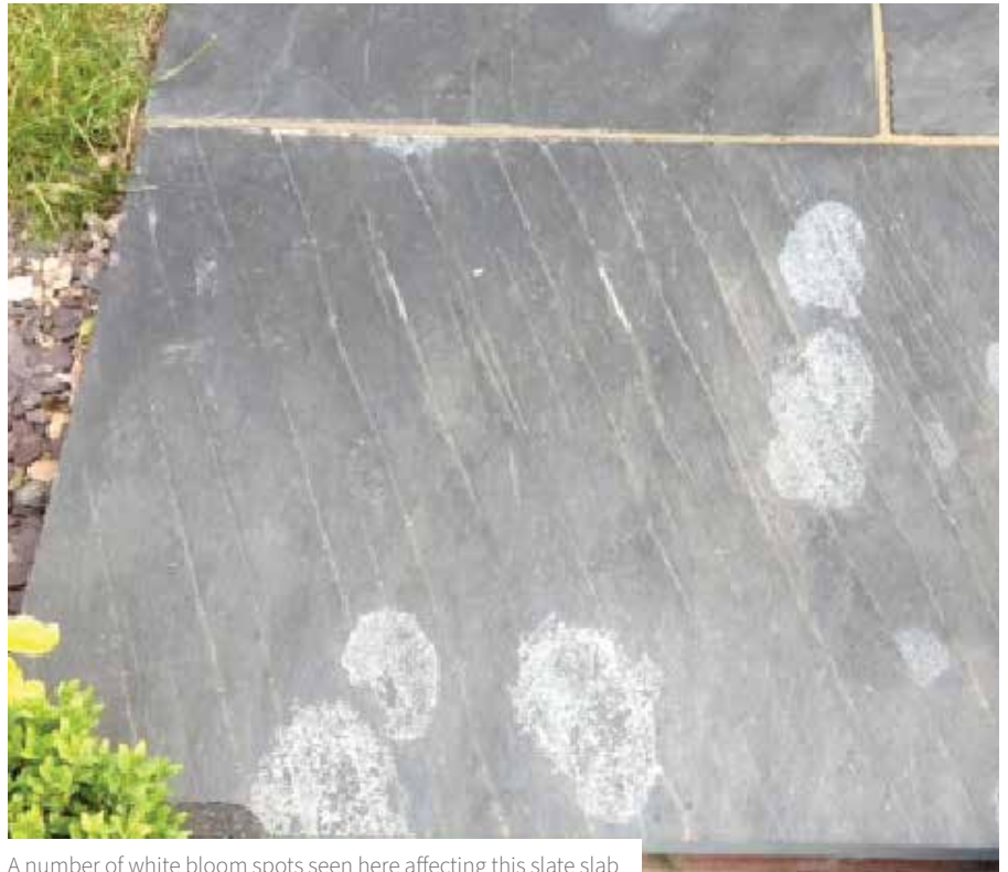
A number of white bloom spots seen here affecting this slate slab
