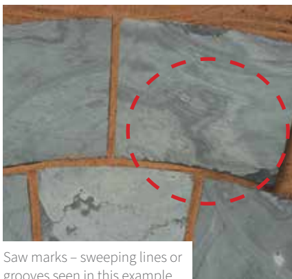
The white marks seen here are characteristic signs of saw marks
