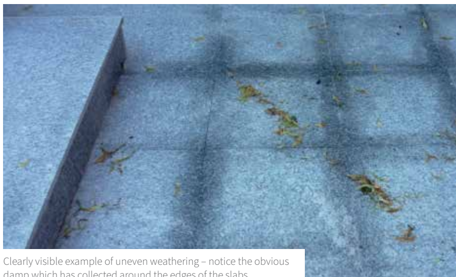
Damp patches around some of the joints are visible in this example
