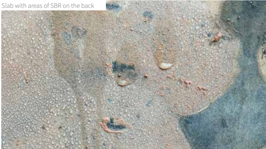
Slab with areas of SBR on the back
