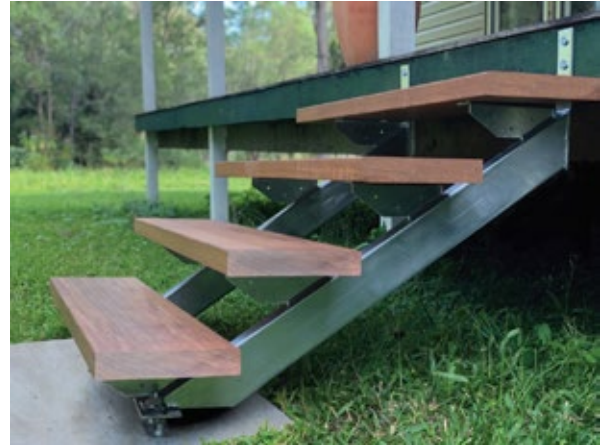
4T-SSBD installed with Merbau Treads.
