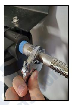
**NOTE:** If pipe fittings are used, be sure to use Teflon tape on the threads prior to installing the fitting on the filter housing. If copper pipe and fittings are being used, make sure all solder joints within 12-15' of the filter housing are completed and the pipe is cool, prior to connecting it to the housing fittings.
