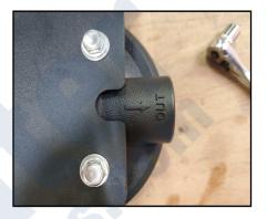
3. Install threaded nipples or other threaded fittings in the housing. Be sure to use Teflon tape on the fittings. Tighten them with a pair of channel locks. If flex pipes with rubber gaskets are used, there is no need to Teflon tape the outer fittings. If a normal plumbing fitting is used, then be sure to Teflon tape the outer fitting.
