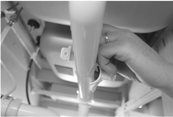
Drain saddle valve installation
