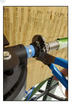
**NOTE:** If pipe fittings are used, be sure to use Teflon tape on the threads prior to installing the fitting on the filter housing. If copper pipe and fittings are being used, make sure all solder joints within 12-15' of the filter housing are completed and the pipe is cool, prior to connecting it to the housing fittings.
