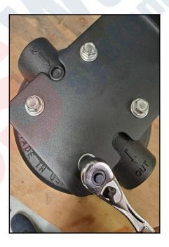
3. Install threaded nipples or other threaded fittings in the housing. Be sure to use Teflon tape on the fittings. Tighten them with channel locks. If flex pipes with rubber gaskets are used, there is no need to Teflon tape the outer fittings. If a normal plumbing fitting is used, then be sure to Teflon tape the outer fitting.
