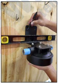
5. Shut off the water and release the water pressure at the lowest sink or spigot. Cut the pipe and connect it to the filter. Connect the inlet plumbing to the inlet on the filter housing. Tighten with channel locks.
