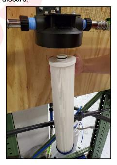
5. Lubricate the O-rings and install the new filter in the filter housing cap.
