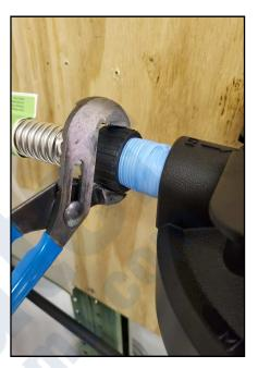
6. Connect the outlet plumbing to the outlet on the filter housing. Tighten with channel locks.
