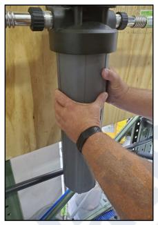
NOTE: The housing should spin tight fairly easily. If not, add more lubrication to the sump threads. This will aid with removing the sump when the filter needs to be replaced again.
