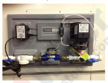
3. Now install the inlet plumbing from the sediment filter to the left side of the injection panel. Use the 3/4" Union Adaptors to connect to the panel. These adaptors are designed for 3/4" PVC. If 1" plumbing is used the 1" x 3/4" Bell Reducers can be used to adapt the 3/4" Union Adaptors to 1" connections. A small piece of 3/4" pipe is needed to connect the 1" x 3/4" Bell Reducers to the 3/4" Union Adaptors.
