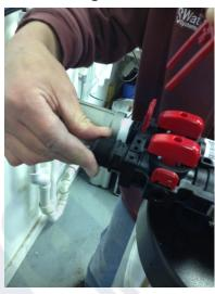
6. Attach the inlet and outlet plumbing to the control valve. Be sure to check the stamped arrows on the valve and bypass for inlet/outlet orientation.
