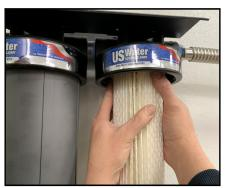
NOTE: The radial flow carbon filter is installed in the first position and the Limeblaster in the second position.
