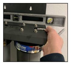
5. Shut off the water and release the water pressure at the lowest sink or spigot. Cut the pipe and connect it to the filter. Connect the inlet plumbing to the inlet on the filter housing. Tighten with an adjustable wrench.
