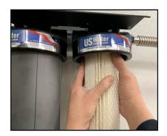
8. Lubricate the O-ring on the filter housing sump and install it. Tighten the filter sump hand tight. That should be adequate. Do not use abrasive tools to tighten the housing or damage may occur.
