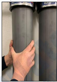
NOTE: The filter will fit tightly in the housing cap. It will take force to push the filter in the cap. This ensures a positive seal. Be sure the filter is pushed all the way in the cap.
