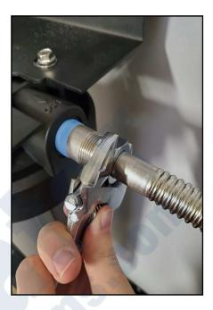
**NOTE:** If pipe fittings are used, be sure to use Teflon tape on the threads prior to installing the fitting on the filter housing.
