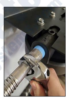
6. Connect the outlet plumbing to the outlet on the filter housing. Tighten with an adjustable wrench.
