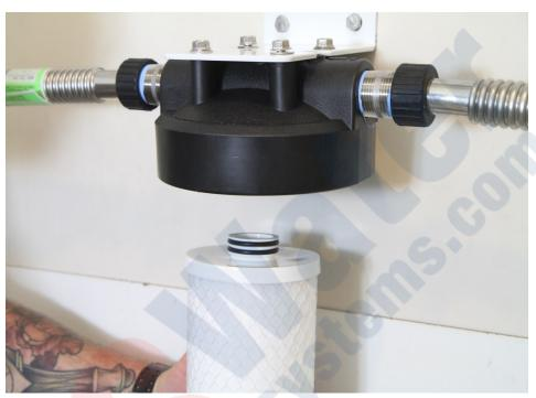
7. Lubricate the O-rings and install the new filter in the filter housing cap.
