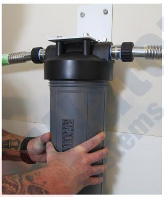
NOTE: The housing should spin tight fairly easily. If not, add more lubrication to the sump threads. This will aid with removing the sump when the filter needs to be replaced again.
