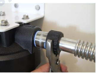
do not require Teflon tape. If pipe fittings are used be sure to use Teflon tape on the threads prior to installing the fitting on the filter housing. If copper pipe and fittings are being used make sure all solder joints within 12-15" of the filter housing are completed and the pipe is cool, prior to connecting it to the housing fittings.
