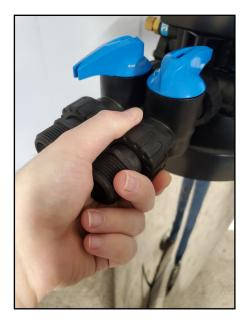
5. Be sure to use Teflon tape or other pipe sealant on the plumbing fitting threads and install them on the bypass accordingly. Use an adjustable wrench to ensure they are tight.
