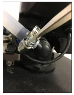
NOTE: Be sure to secure the drain line. The softener will drain with force and it should be secured to prevent a leak. Hose clamps should be used to secure the drain line at the connection points.
