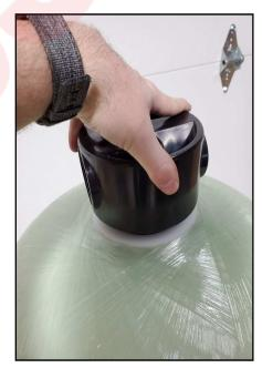
8. Install plumbing fittings into the inlet of the in/out head. Be sure to use Teflon tape on the fittings. Tighten them hand tight then, using a pair of channel locks, tighten an additional 1/4 turn.
