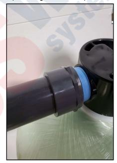
10. Install plumbing fittings into the outlet of the in/out head. Be sure to use Teflon tape on the fittings. Tighten them hand tight then, using a pair of channel locks, tighten an additional 1/4 turn.
