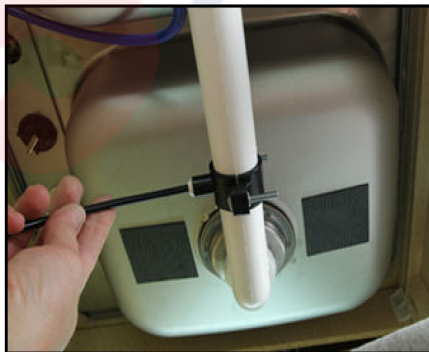
Drain saddle valve installation
