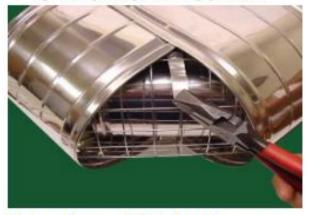
Using pliers, pull Tab A until screen tightens against inside of outer hoods.
