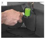
First of all, stretch the moulded part (tongue) in the corner areas (top and bottom) (see shaded areas). Then place the tongue over the inverted pleat at a distance of 3 mm above the roof waterproofing membrane and fully surface-weld.
