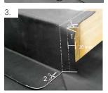
Cut 20 mm into the top projection (1.) and cut into the bottom projection as far as the corner (2.). Form an inverted pleat.
