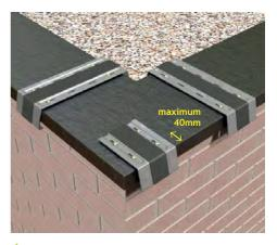
4. Always secure additional half brackets for corners and piers with the first fixing point with a maximum of 40mm from the external wall finish.
