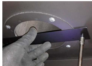
Figure 8.b.c Restrictor plate Installation
