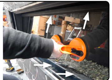
Figure 21.b Installing the door
