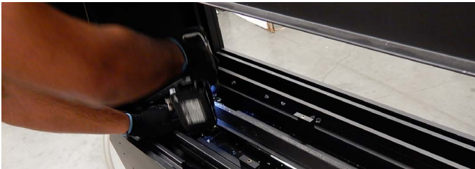
Figure 12.d Removing the Burner screws
