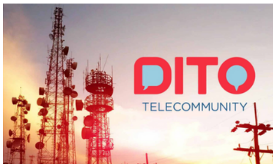
Dito Telecommunity Various Cell Sites
