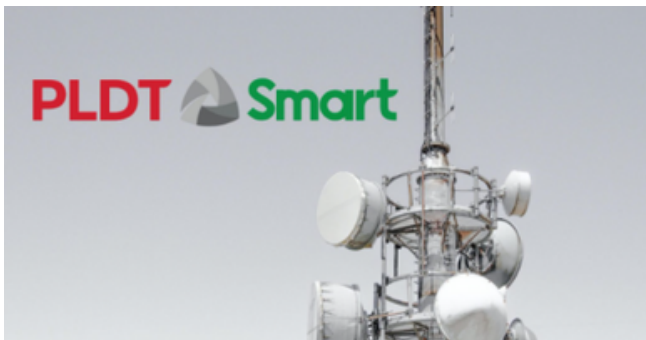
PLDT and Smart Telecom Various Cell Sites
