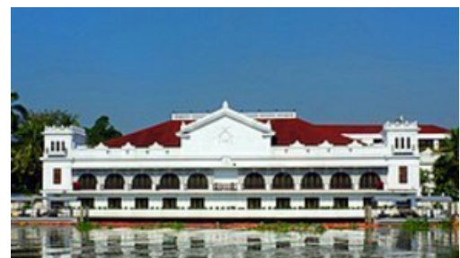
Malacañang Palace Kitchen and Office
