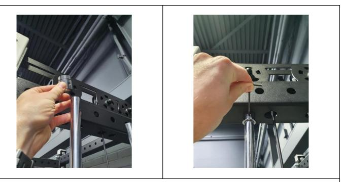
9. Reinstall the Guide Rod Locks by sliding the Guide Rod Locks on to the Guide Rods.
