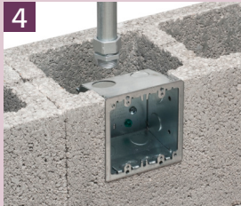
Install the EMT in the top of the box. Top view: EMT installed in box.
