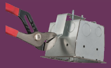
Install the EMT in the top of the box. Top view: EMT installed in box.
