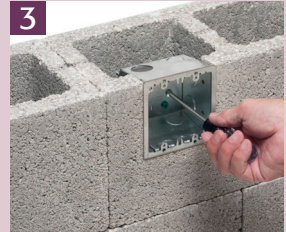
Tighten the screws on the spring clip to pull it securely against the block.
