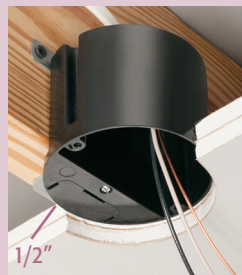
Set-back in double drywall
