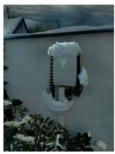
Snow and ice accumulating on the charging station make it uncomfortable to use, if not completely obstructing plugs and controls.
