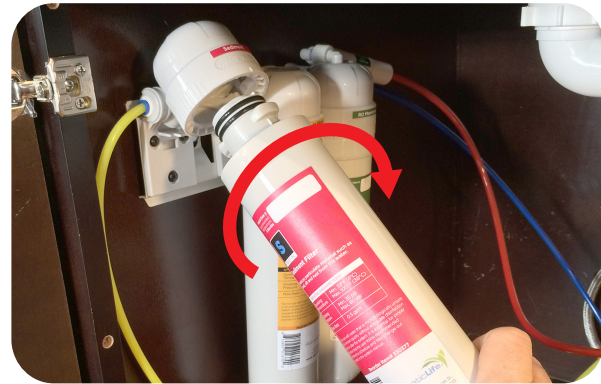
Install: Twist right
