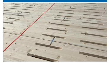
Align ADHERO VISTO with the marking. Plan the installation such that there is continuous adhesion with a flat surface.
