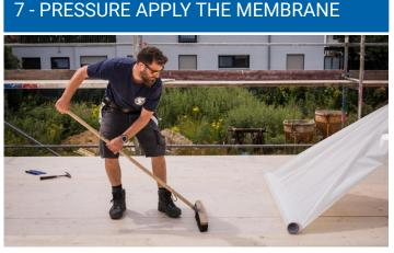
Press the membrane firmly into place using a PRESSFIX XL application tool, broom, or roller.
