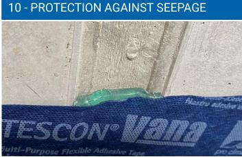
Any gaps or defects are to be covered with TESCON VANA in a waterproof manner or, filled with CONTEGA HF.
