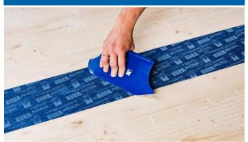
As an alternative method, the membranes can be taped to one another using TESCON VANA 100. Position the tape centrally and gradually stick it in place with no folds or creases. Ensure a minimum of 2" (100mm) adhesion to both membrane substrates. Pressure apply using the PRESSFIX XL.
