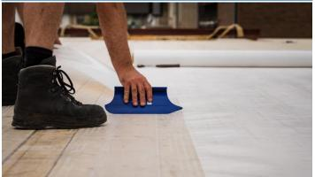
Remove the 10" (250mm) adhesive strip. Pressure apply the membrane firmly into place using the PRESSFIX XL application tool, broom, or roller.
