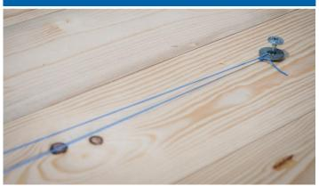
Mark a line on the CLT to position the first ADHERO VISTO edge to be applied.
