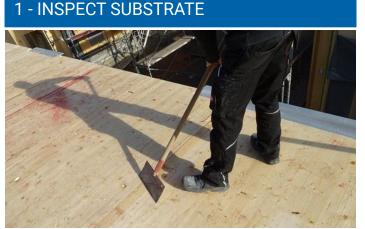
Clean dirt, debris and remove any protruding elements (splinters, nails, screws, etc) that can damage the membrane during installation.
