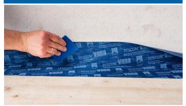
Pretreatment with TESCON PRIMER RP is necessary for CMU, masonry, and concrete. When in doubt, verify adhesion with an adhesion test. For very rough substrates and for joining vertical elements/shafts, it is recommended to use CONTEGA HF and TESCON VANA to ensure complete waterproof connections. For vertical interruptions (walls, elevator shafts), the minimum vertical height should be 4-6" (100-150 mm).
