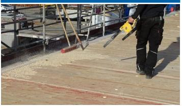
Make sure the substrate is clean. Use compressed air or a blower to clear dirt and debris. Remove any oil, silicone or grease that would prevent proper adhesion of the membrane.
