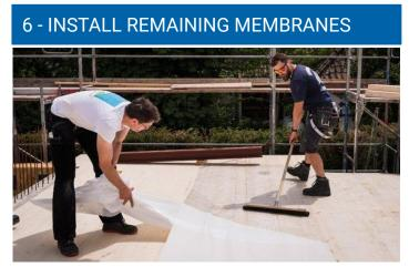
Remove the remaining release paper. Press the membrane firmly into place using a PRESSFIX XL application tool, broom, or roller.
