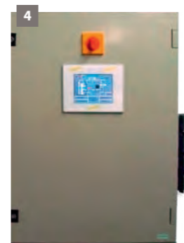
1 | Auto-pump 2 | PLC screen 3 | Measurement screen 4 | Automatic management cabinet 5 | Posibox
