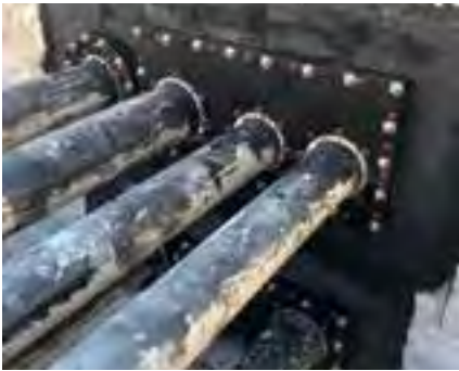
KRASO® Plastic Flange Plate Type KFP multiple with foil flange - Special for the installation of media lines using KRASO® Sealing Insert in front of a core drilling in concrete or masonry wall, plate made of 60 mm thick, high-strength special plastic, with EPDM flat seal, fixing and sealing material and PU 50, 1 x 250 mm, 2 x 215 mm KRASO® Special Sealing Inserts Type SD40-T non-corrosive stainless steel V2A / 40 mm seal MPA-tested up to 3 bar, for KFP: 249 mm, media line: 203 mm, for KFP: 214 mm, media line: 166 mm
