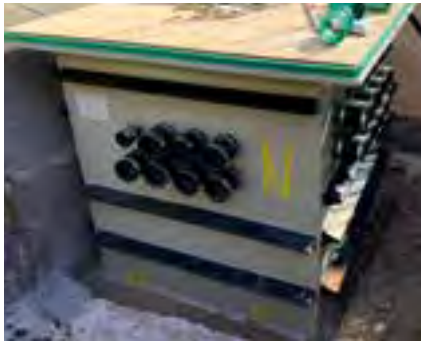
KRASO® Pump Sump Type Q - Special with 15 cm surrounding fixed-flange and water pressure tight surrounding KRASO® 4 Seal on the fixed flange, reinforcing ribs and concrete anchors and 35 water pressure tight KG pipe connections internal dimensions: approx. 145 x 170 x 135 cm total weight: approx. 290 kg
