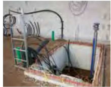
KRASO® Pump Sump - concrete - Special internal dimensions approx. 250 x 150 x 120 cm, 3 x KRASO® Cable Penetration KDS 150 on one side package 1 x 3, KRASO® Casing Type FE ID 200 on one side with welded sleeve, made of waterproof concrete, with 20 cm thick, reinforced wall and base plates ( 20 kg/ per cbm ), rebar connection approx. 8/15 two-rowed, surrounding water pressure tight, MPA-tested construction joint tape KRASOflex® Duo-Fix 150 „plus“, 4 lifting lugs Rd30, weight/piece: approx. 7.8 t
