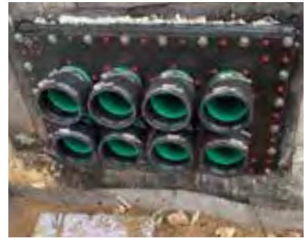
KRASO® Plastic Flange Plate Type KFP 150 Multiple 2x4 8 x 160 mm with welded KG 2000 spigot for the connection of a hose connection (10 cm protrusion length) MPA-tested up to 3 bar, plate made of 60 mm thick, high-strength special plastic, with EPDM flat seal, fixing and sealing material and PU 50, wall opening incl. chamfer strip : 930 x 550 plate size external = approx. 1090 x 710 mm
