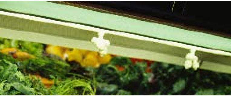
Scale buildup in pipes without scale prevention
