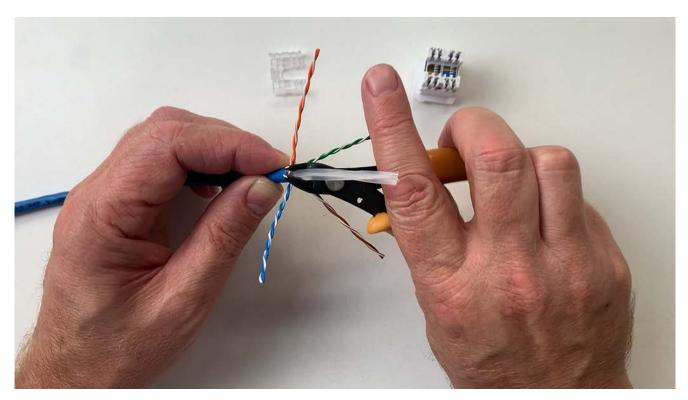
**STAGE 6.**Arrange the 4 pairs based on the required locations on the jack module and untwist the pairs.
