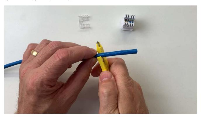
**STAGE 2.**Remove the outer sheath.
