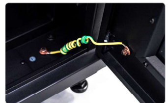
Earth straps on front and rear doors
