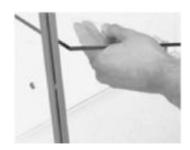
13. Finally, add stability to the glass panels by inserting the rubber seal (R) into the channels where the glass meets the aluminium
