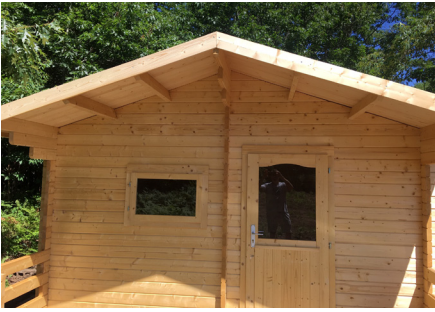
41. View of sauna after fascia boards attached.
