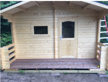
43. View of completed porch.
