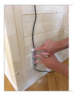
**STEP 6** - Mount the power supply to the exterior sauna wall, ceiling or other place where you can secure with either screws or small nails (not included). Plug the power supply into a 110v outlet and turn on the On/Off LED switch.
