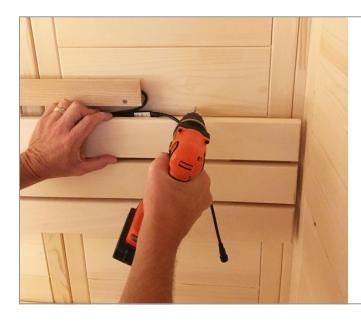
**STEP 3** - Locate where you want the cord to exit the sauna. Drill a 5/8" hole through the sauna wall
