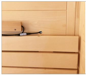
**STEP 4** -Feed the power cord coming from the LED bar through the hole so that the power switch remains in the sauna.
