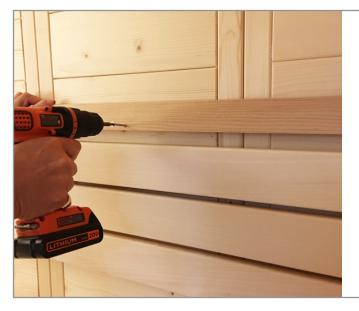
**STEP 2** -Level the LED bar and attach to the sauna wall using the screws provided
