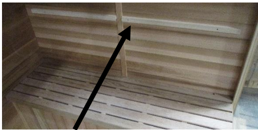
Wood Plank on REAR WALL PANEL
