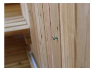
a. For barrel saunas, the 1 1/2" lag screws should be mounted approximately 20" off the lowest point of the barrel and spaced 15 1/4" apart and centered above the vent holes. Note: The heater will conceal a portion of the LED light. This is normal.
