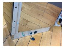
**NOTE:** While this location is the most common, the power can enter the sauna at any location. It is not recommended you use the predrilled vent holes as an entrance for the conduit.
