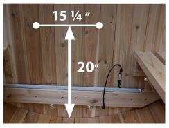
**b. For indoor saunas**, the screws should be mounted 20" off the floor, and spaced 15 1/4" apart approximately centered above the vent holes (if present). It is fine that the heater is covering the holes as ventilation still occurs.
