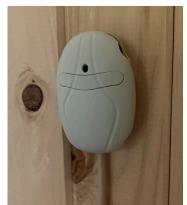
Next, feed the sensor wire out of your sauna in order to connect to the power unit.
