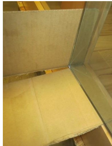
Cardboard placed vertically & horizontally between glass door and door jamb
